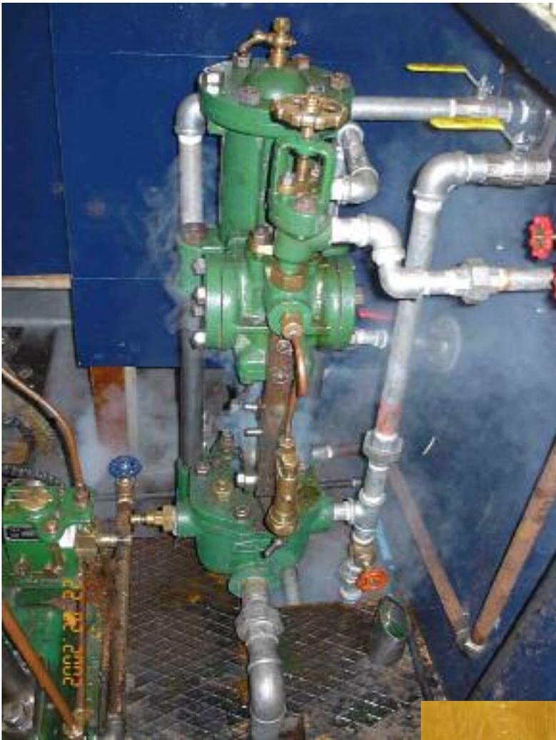
The Weir pump sitting to the left of the engine when facing the rear of the boat. All the pipe work still requires lagging and painting
