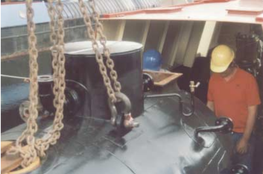
Craning the boiler in onto greased slides
