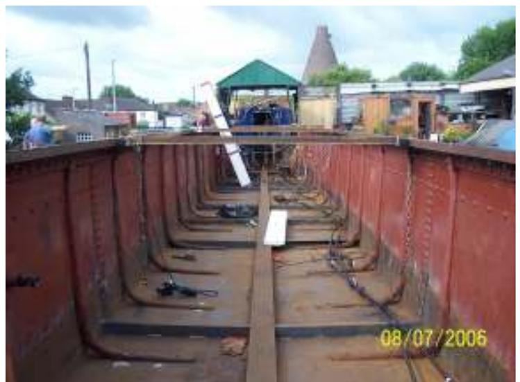
The boat's bottom and footings soon fell foul of the oxy-propane torch and a large amount of rust, scale and steel was soon pulled and swept out from under the boat. A lot of hammering of the knees resulted in one or two becoming detached from the sides as the rivets fell out! Regrettably some very thin spots were found behind the knees and in the front bulkhead of the aft cabin.
