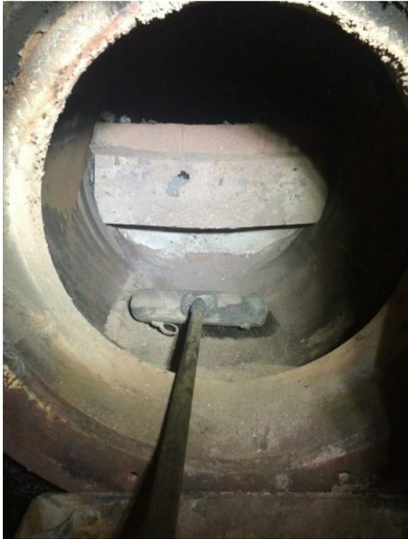
*Left - Nice and Clean! looking in at the back of the boiler, in the back ground you can see the brick wall that is at the back of the firebed.*
