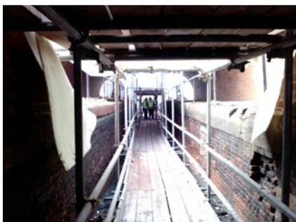
There was a walkway laid all along the canal bed under the bridge to the other end of the lock. The state of the brickwork was visible along both sides of the lock. It was apparently worse than expected and the stoppage was going to be extended until the 21st.
