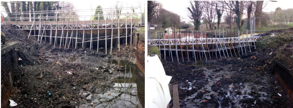
Fabric dams had been placed across the canal (above left - north side, right - south) at either end of the lock and you could see why we had run aground so often. Dredging on the approaches to the lock were not part of the planned work, but we were told that one of CRT's dredgers would be passing through here next year and it would be done then.
